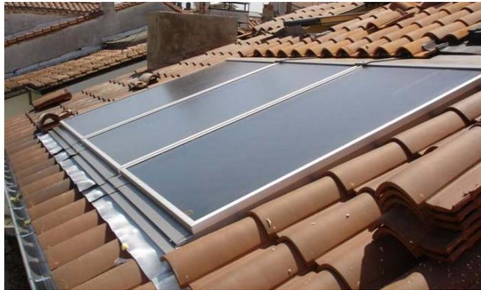
Figure - Example of a solar thermal system integrated in a historical area roof.
